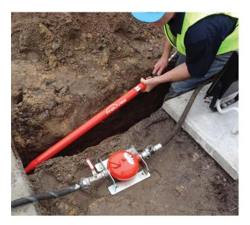
PneuVibe offers two alternative head designs for the earth piercer depending upon varying soil conditions.
